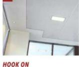
Fully demountable. Available in different sizes, perforations and colours. Used with mineral wool pads to achieve different thermal and acoustical specifications.
